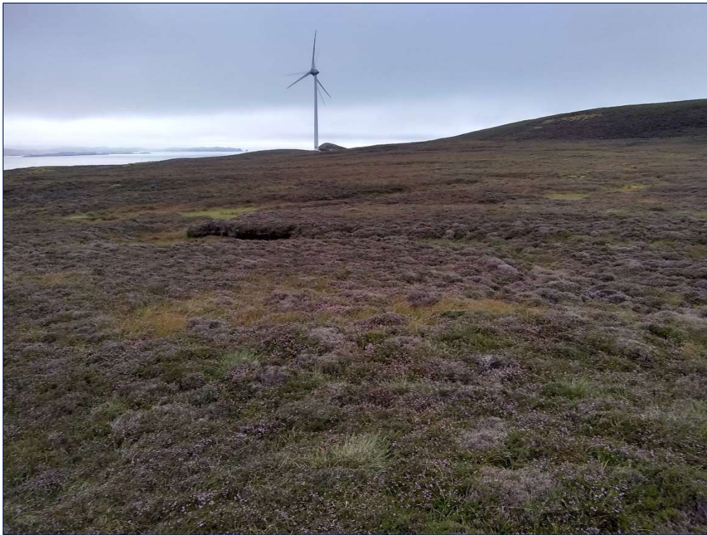
Plate 12-1: North facing view of the Operational Turbine (T1) on the site
